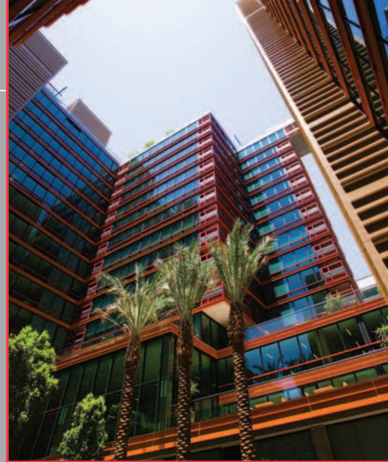
The striking design of Optima Biltmore Towers serves as the new home of Optima’s Arizona corporate headquarters.
